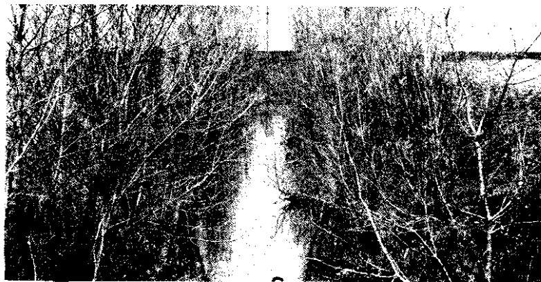
Kaskaskia Mutual Dredged Channel near Bondville, Illinois. Approximate bottom width 10 feet. Picture taken April 1925.
