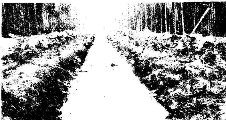
Back Swamp Dredged Channel near Lumberton, North Carolina. Approximate bottom width 15 feet. Picture taken in 1915.
