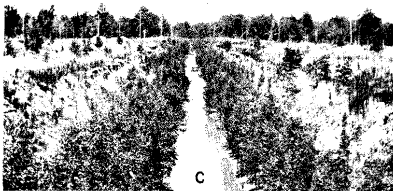
Cummins Lake Dredged Channel near Gould, Arkansas. Approximate bottom width 30 feet. Picture taken June 1926.
