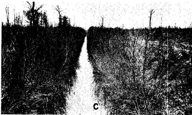
Ditch No. 1 of Little River Drainage District near Chaffee, Missouri. Approximate bottom width 10 feet. Picture taken December 1925.
