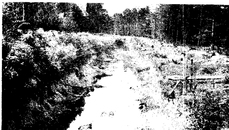
Sugar Creek Dredged Channel near Henderson, Tennessee. Approximate bottom width 15 feet. Picture taken 1917.
