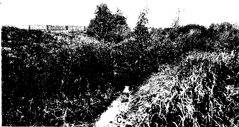
Stewart Branch Dredged Channel near Champaign, Illinois. Approximate bottom width 15 feet. Picture taken October 1926.
