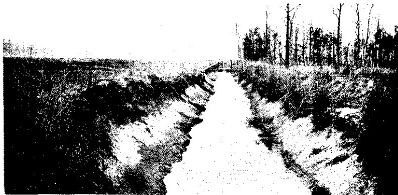
Chawappah Creek Dredged Channel near Shannon, Mississippi. Approximate bottom width 15 feet. Picture taken 1913.
